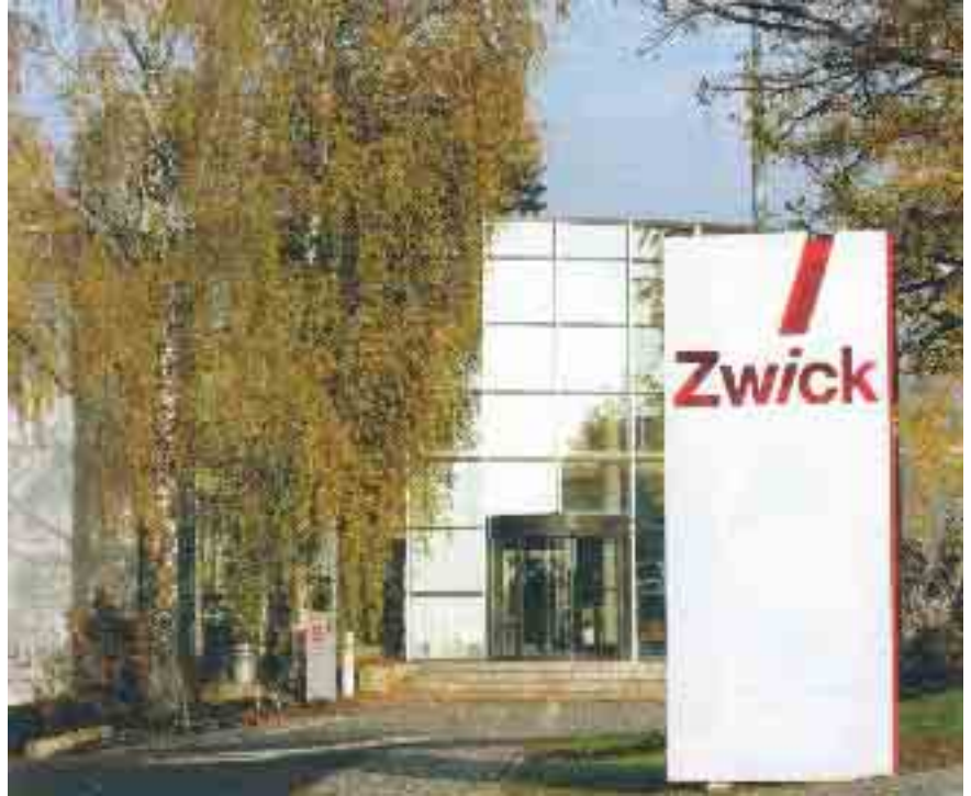
Headquarters of Zwick Roell AG and Zwick GmbH & Co. KG at Ulm, Germany
